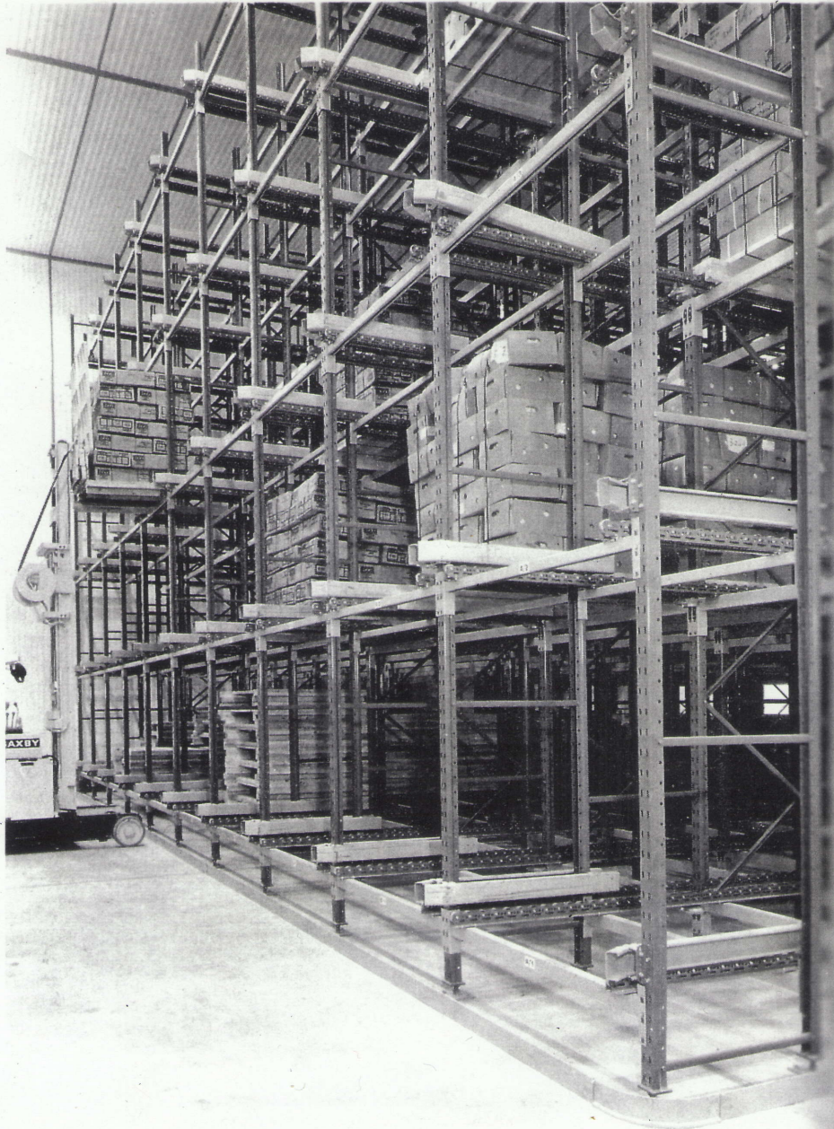
10 Live storage of palletised loads ( By courtesy of Dexion Ltd. )
